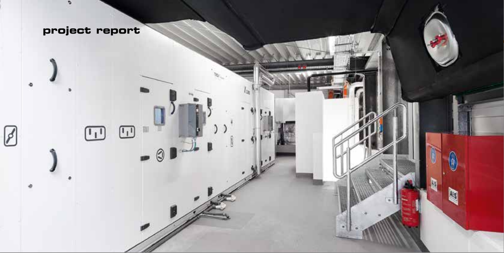
X-CUBE air handling unit for a volume flow rate of 22,000 m 3 /h.
