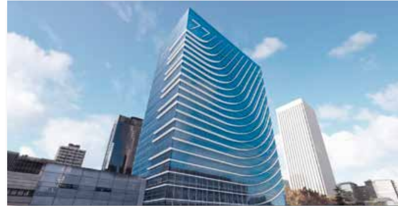
Castellana 77 office and apartment complex, Madrid, Spain: More than 5000 induction units
