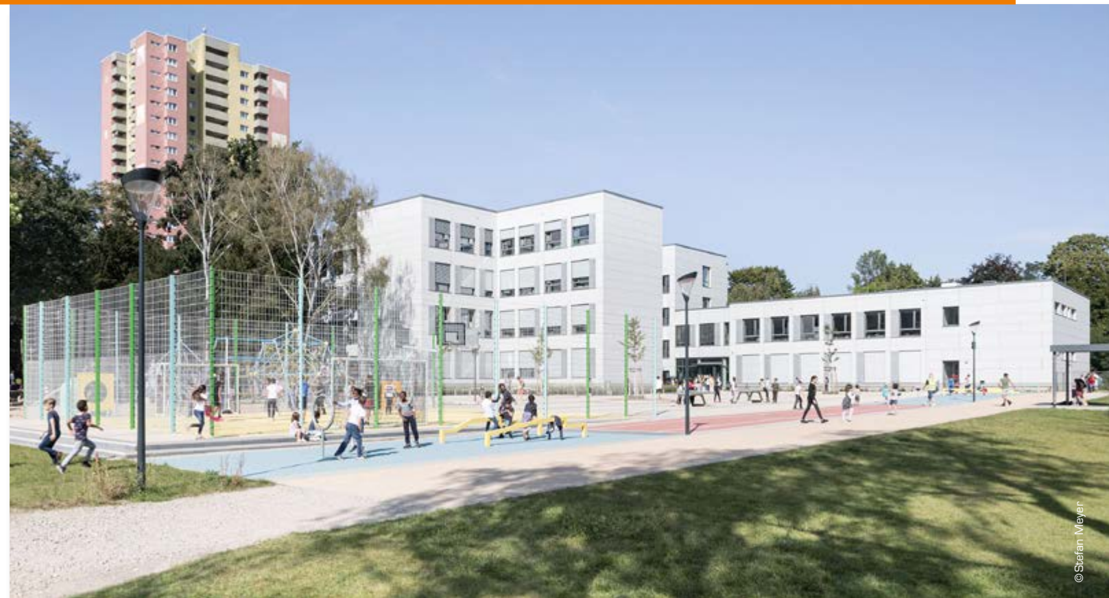
The Marienfelder Grundschule primary school was refurbished from the ground up and equipped with modern ventilation units.
