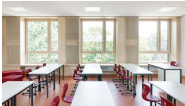
Facade-integrated ventilation units provide sufficient air exchange and healthy air in the classrooms.
