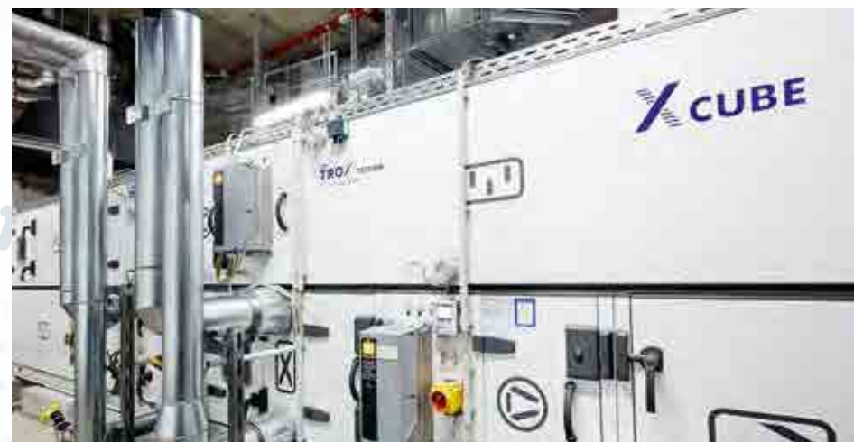
A total of 30 X-CUBE air handling units provide 450,000 m 3 /h of treated fresh air to GERBER.
