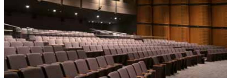
Lecture theater in Dubai, with TROX diffusers installed in the steps
